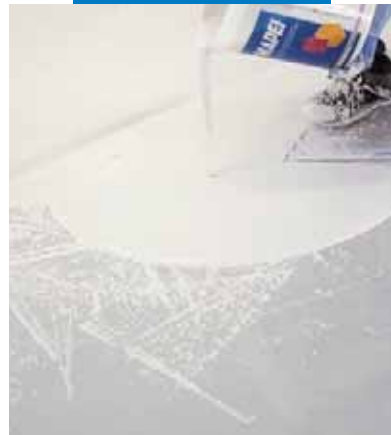
Manual application of Ultratop
