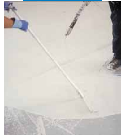
Mechanical application of Ultratop
