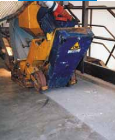
Preparation of the substrate by peening
