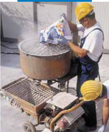
Mechanical preparation of the product before pumping
