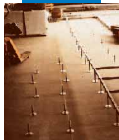
Slab levelled with Ultraplan ready for fixing a floating floor
