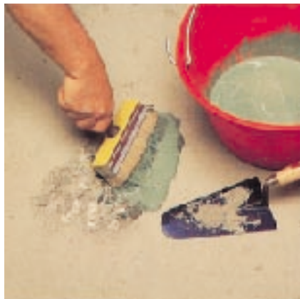
Floor patching: application of slurry
