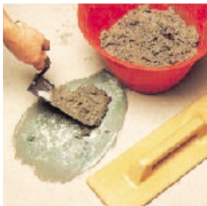
Floor patching: application of mortar
