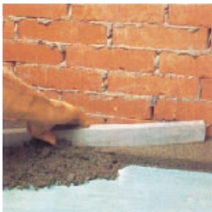
Applying adhesive cement screed modified with PLANICRETE
