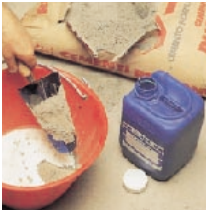
Mixing cement mortar with PLANICRETE
