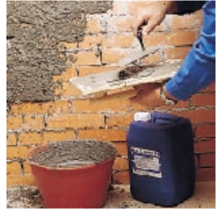
Adhesive shotcrete modified with PLANICRETE
