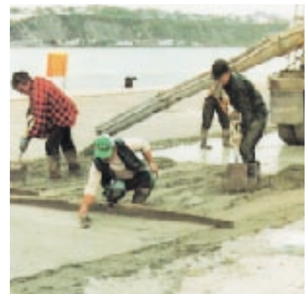
Exterior flooring with concrete admixed with PLANICRETE. Vieux Port, Quebec, Canada
