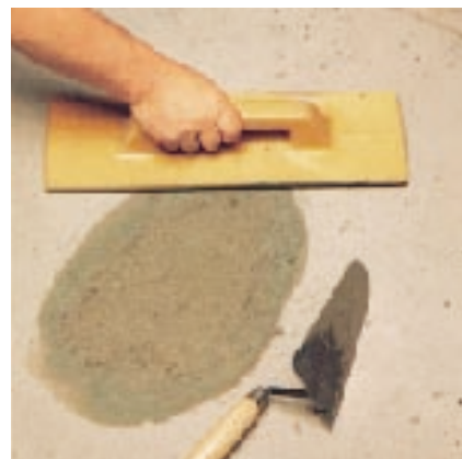
Floor patching: final smoothing
