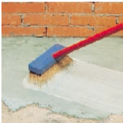
Applying adhesive cement slurry modified with PLANICRETE
