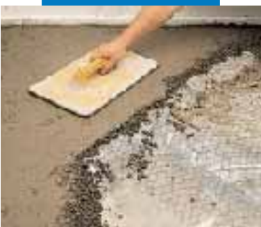
Covering pipes with Mapecem and reinforcement netting
