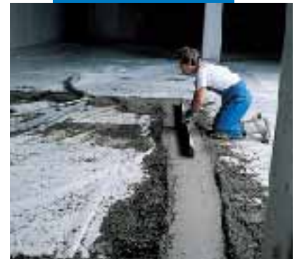
Preparing a levelling strip
