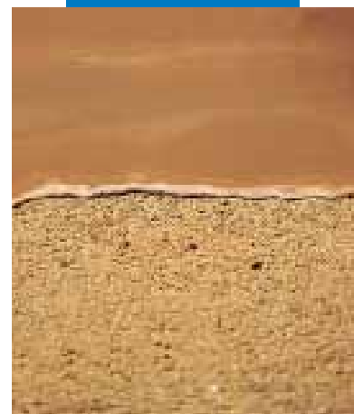
Finishing a Mapecem screed with Ultraplan self-levelling compound
