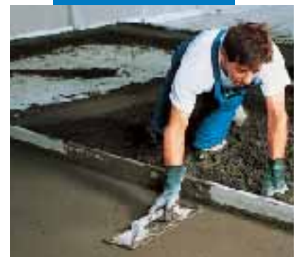
Tamping the Mapecem screed
