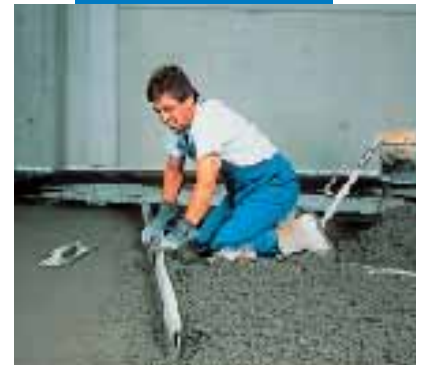
Using the straight-edge
