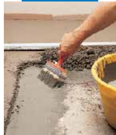
Spreading the anchoring slurry for bonded Mapecem screeds
